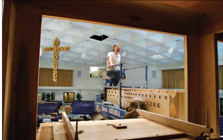
Rising three stories above the church floor, Jeremy Quigley uses a lift to move a heavy wind chest for the new Lively Fulcher organ into place.
